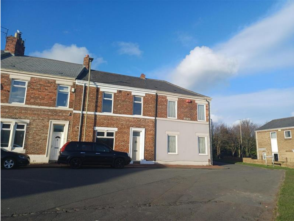
Appendix 6: Site Photos: Front Elevation
