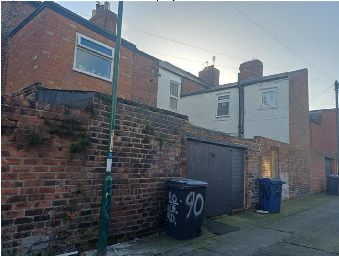
Appendix 7: Site Photos – Rear of Property
